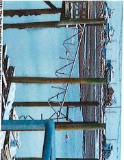
The gangway was partially removed from this location using a crane. However, half of the gangways remains in the water around the northernmost skiff dock area. Removal of this section will be scheduled for this spring before the floats are put back into water. Measurements of the gangway have been recorded, and the process of ordering a new gangway is underway.
